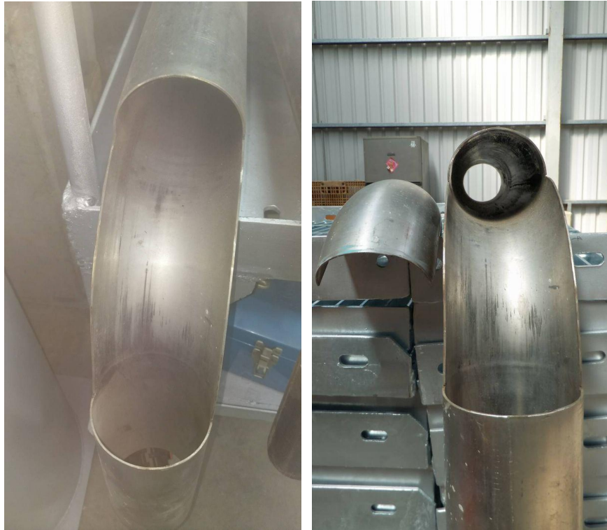
Fig. 3-7: Pipebend slicing, ready for wall thickness measurement (minimum at the center of the pipebend)
